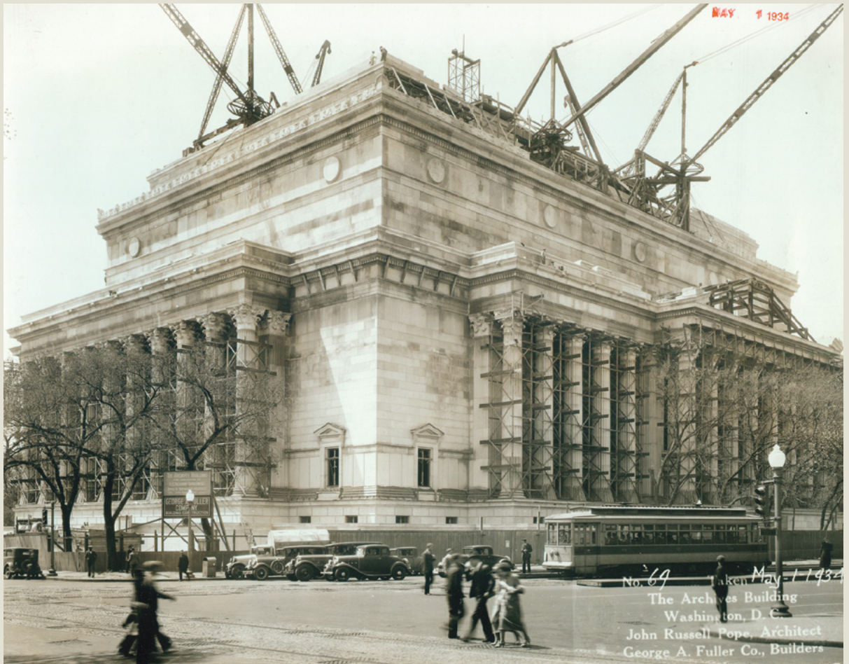
National Archives Building during construction, May 1934.
